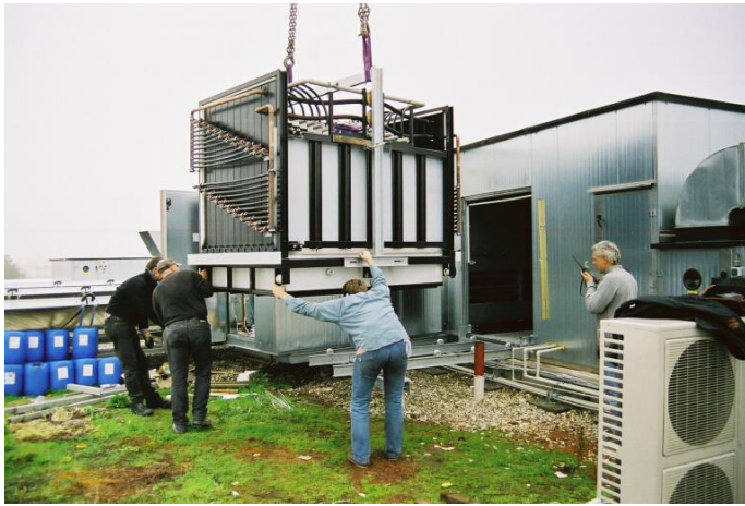
Figure 3: Installation of the dehumidifier
