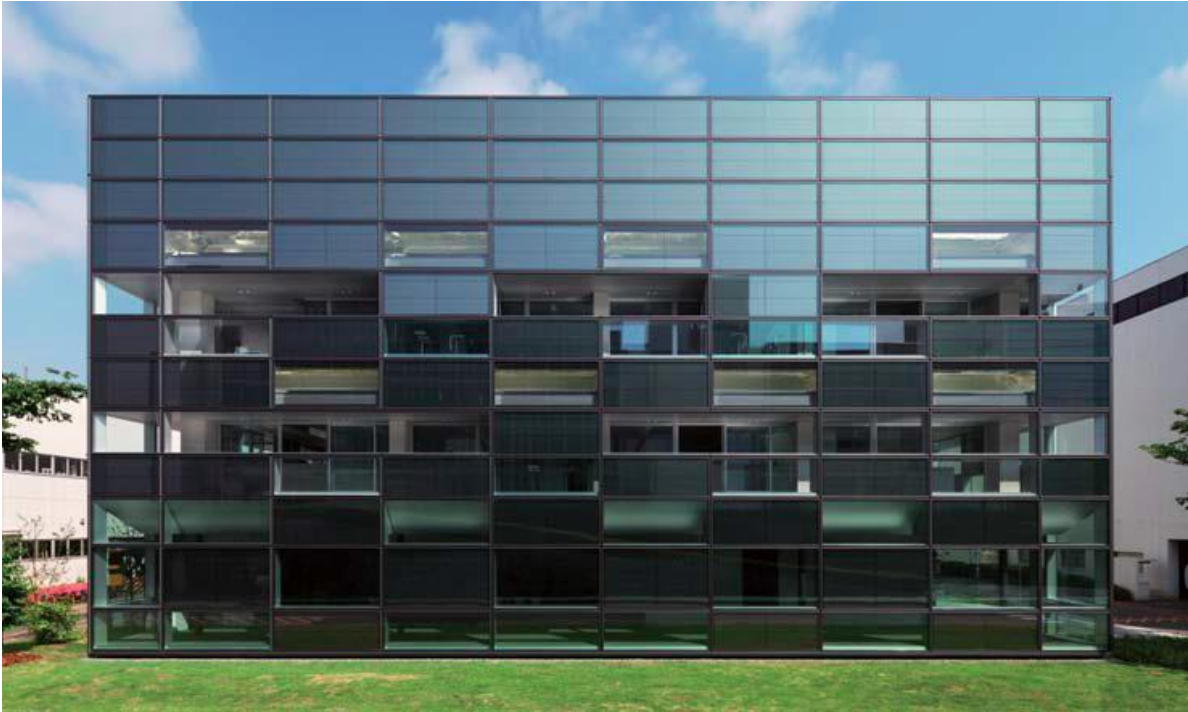
Figure 53: Photovoltaic façade system of Taisei ZEB Demonstration Building.
