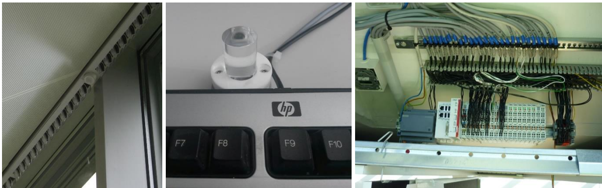
Figure 16: Occupancy sensors between luminaires (left), workplane illuminance sensors (center), and embedded PC in the control cabinet (right).
