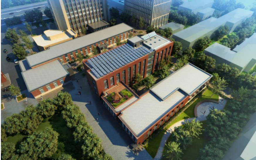
Figure 33: Surroundings of the CABR building.
