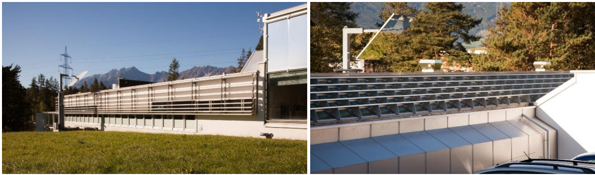
Figure 7: Exterior view of example office with exterior louvers and screen at south façade (left) and sun shading structure at northern pitch roof (right). The heliostat in the right image is used to bring daylight to the basement.
