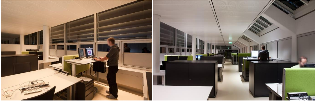
Figure 12: The tunable white electric lighting system provides color temperatures from 2200K to 5000K.
