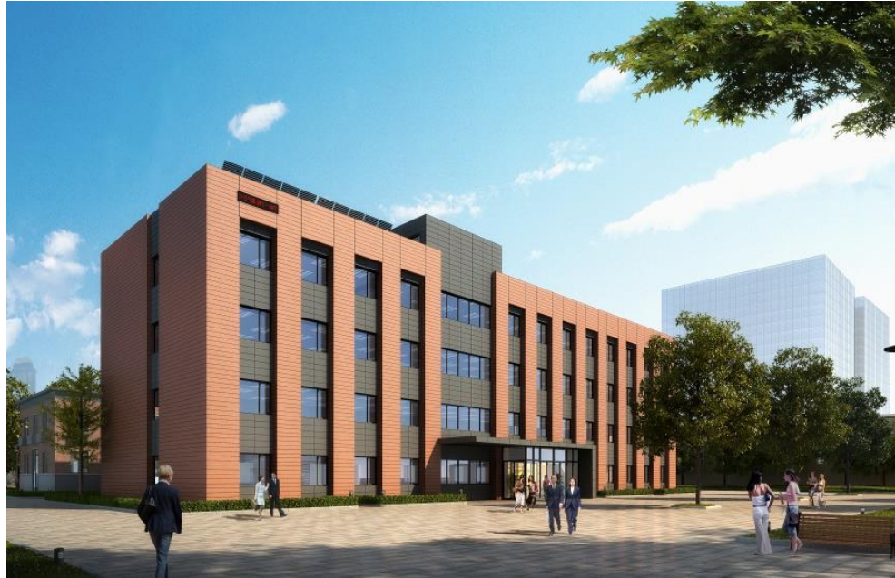
Figure 30: CABR NZEB in Beijing, China.
