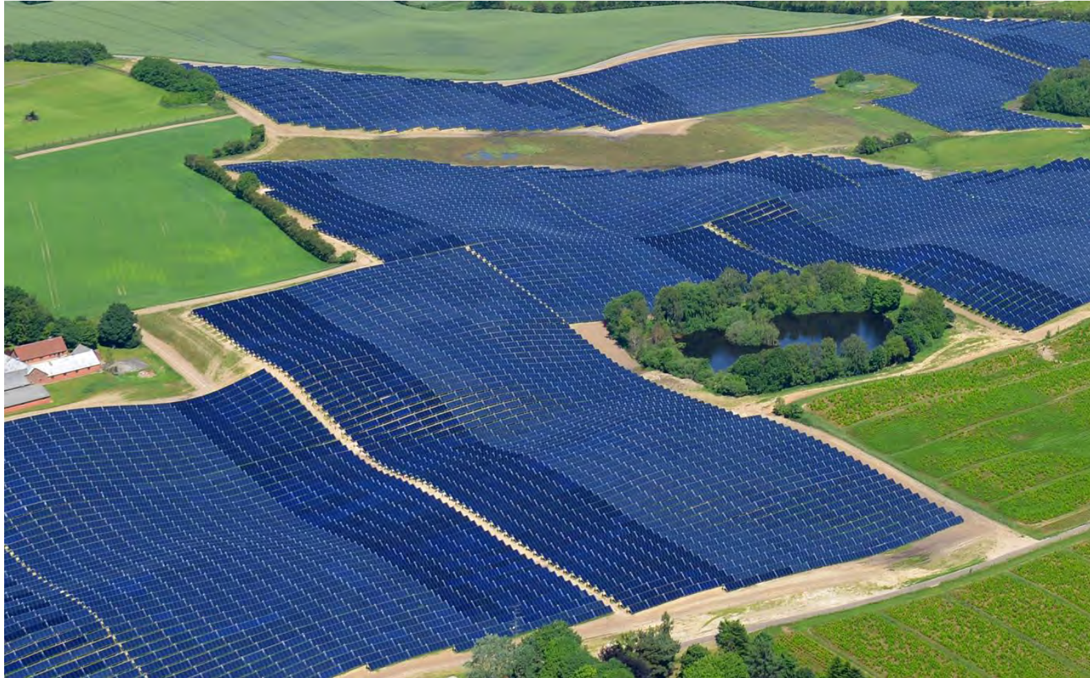
Photo: Arcon Sunmark
