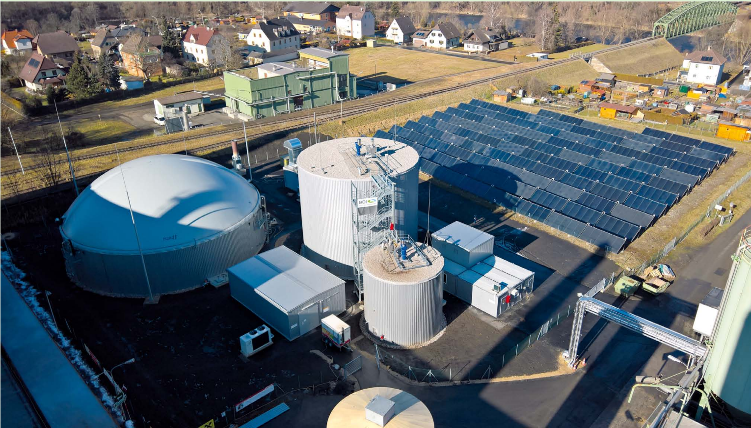
Solar thermal and biogas systems supply the Goess brewery in Austria.
