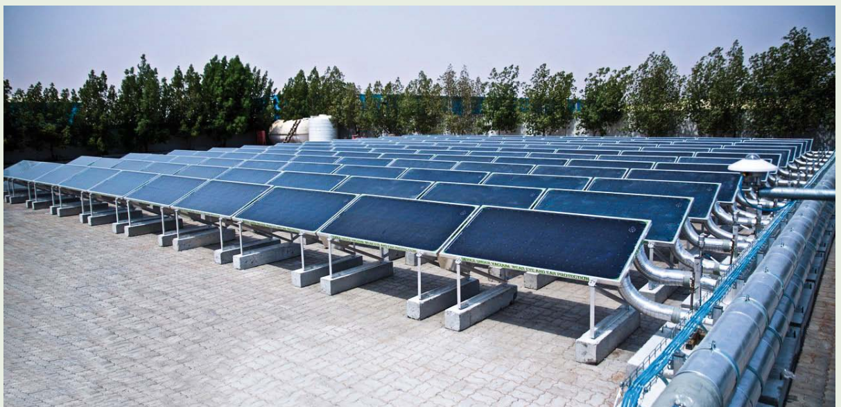
High vacuum flat plat collectors at a rubber factory in Ras Al Kaimah, United Arab Emirates
