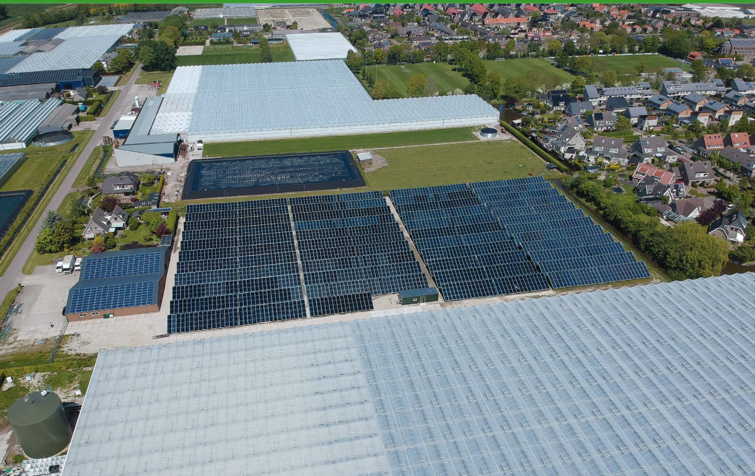
Collector system with 6.5 MW th for heating a greenhouse in Heerhugowaard, Netherlands. The application works as a drain-back system, which means that the collector fluid is water and not glycol.
