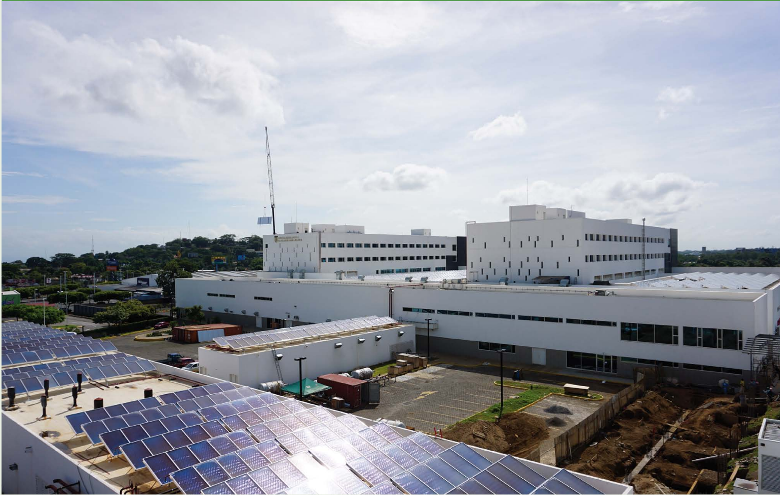
One megawatt of cooling capacity using solar thermal energy at a hospital in Managua, Nicaragua
