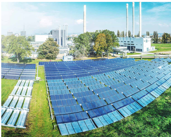
FIGURE 1. Picture of a solar-thermal plant located in Graz, Austria, providing heat for the local district heating network. Copyright: SOLID Solar Energy Systems GmbH.
