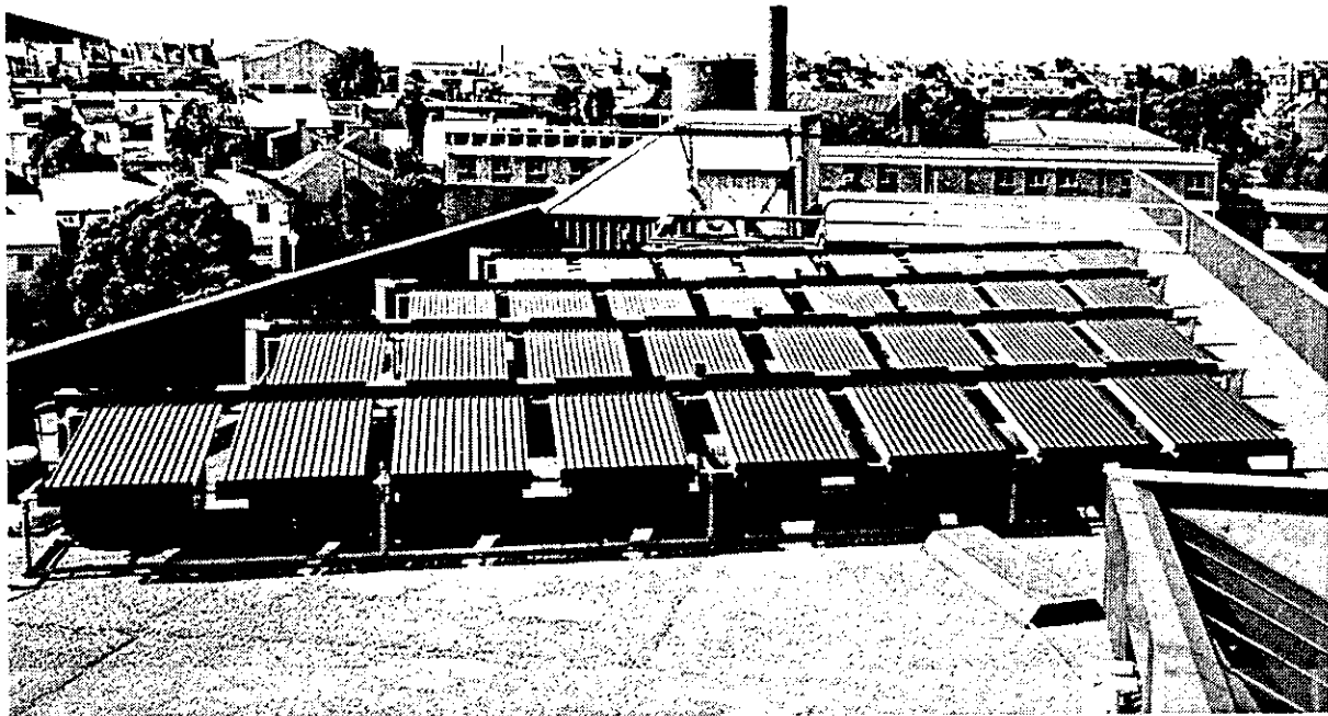
Figure 2-1. Sydney University Solar Heating and Cooling System Sydney, Australia.
