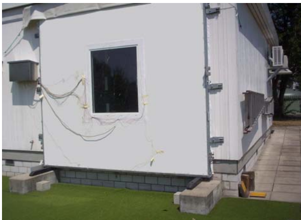
EMPA Test Cells in Duebendorf, Switzerland.
