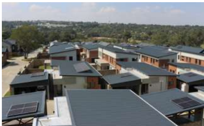
Figure 103. Photovoltaic to heat (PV2Heat) system. Photo: Bongani Xakaza, SANEDI, South Africa
