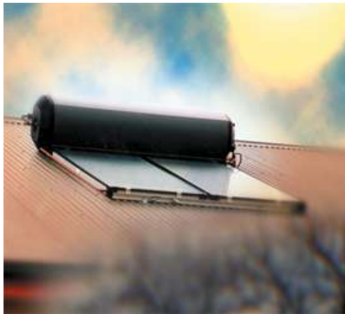
Figure 82. Close-coupled thermosyphon water heater typical for Australia.
