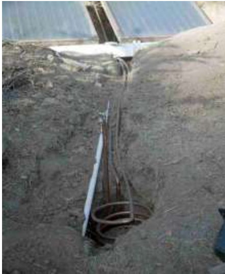
Figure 35. Lower Loop Connects to Buried Coil.
