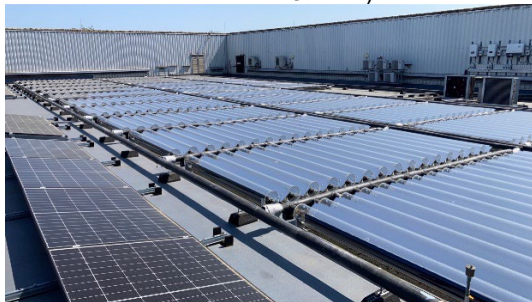
VirtuHOT collectors from Naked Energy sharing roof space with PV modules (Naked Energy. "Westgate Leisure Centre.")
