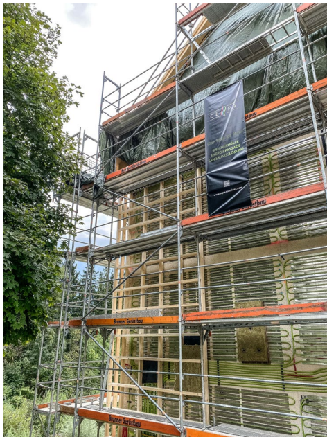
Figure 20: CEPA heating/cooling layer installed on a multifamily house in Austria from Südsan-Project (left) and CEPA system installed in prefabricated façade element for serial renovation (right) source Townern3000
