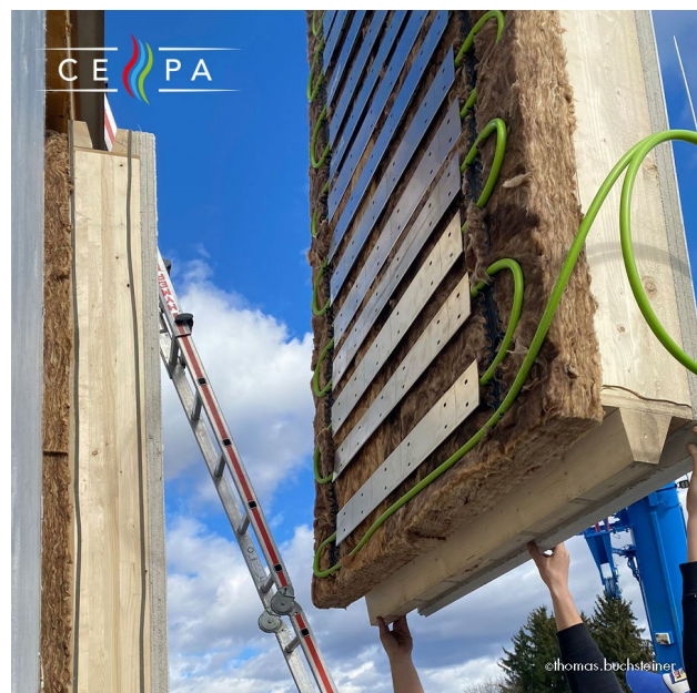
Figure 20: CEPA heating/cooling layer installed on a multifamily house in Austria from Südsan-Project (left) and CEPA system installed in prefabricated façade element for serial renovation (right) source Townern3000
