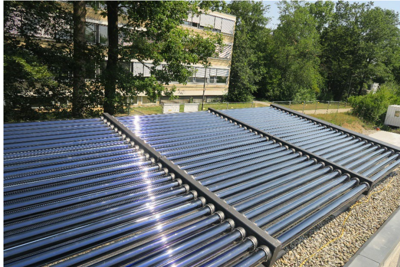
Evacuated tube air collector (airwasol) installed on the roof of the research building at the University of Stuttgart (Source: Institute for Building Energetics, Thermotechnology, and Energy Storage at the University of Stuttgart)
