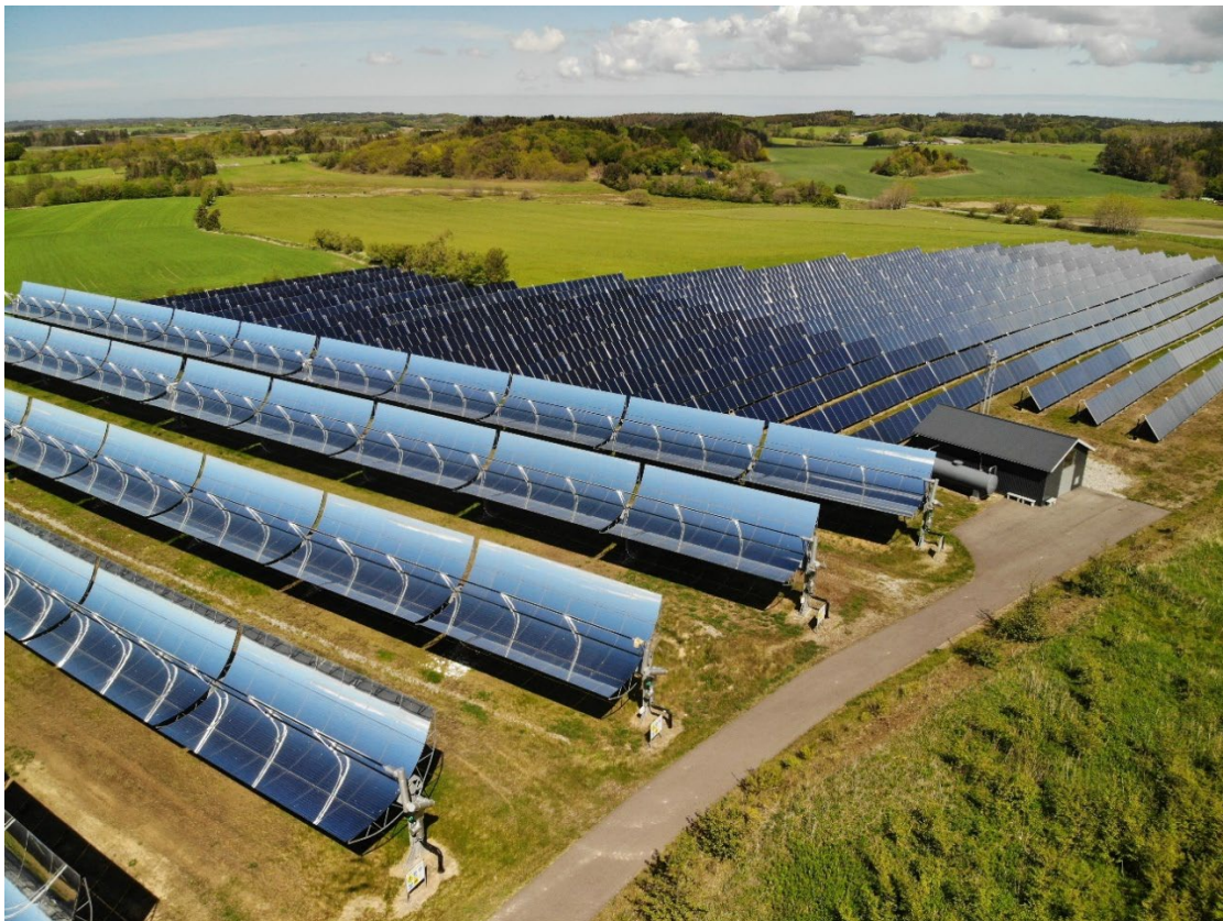
Flat plate collectors with one and two cover plates and one axis tracking concentrating solar collectors at Tårs solar heating plant. (DTU)
