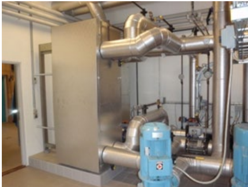
Figure 2. Flat plate heat exchanger. (DTU)
