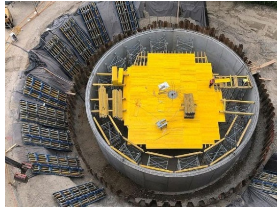
Ice store under construction with a volume of 560 m 3 for supplying heating and cooling to an urban district (Source: https://www.cleantinking.de/eisspeicher-sorgt-fuer-kaelte-und-waerme-im-quartier/ )
