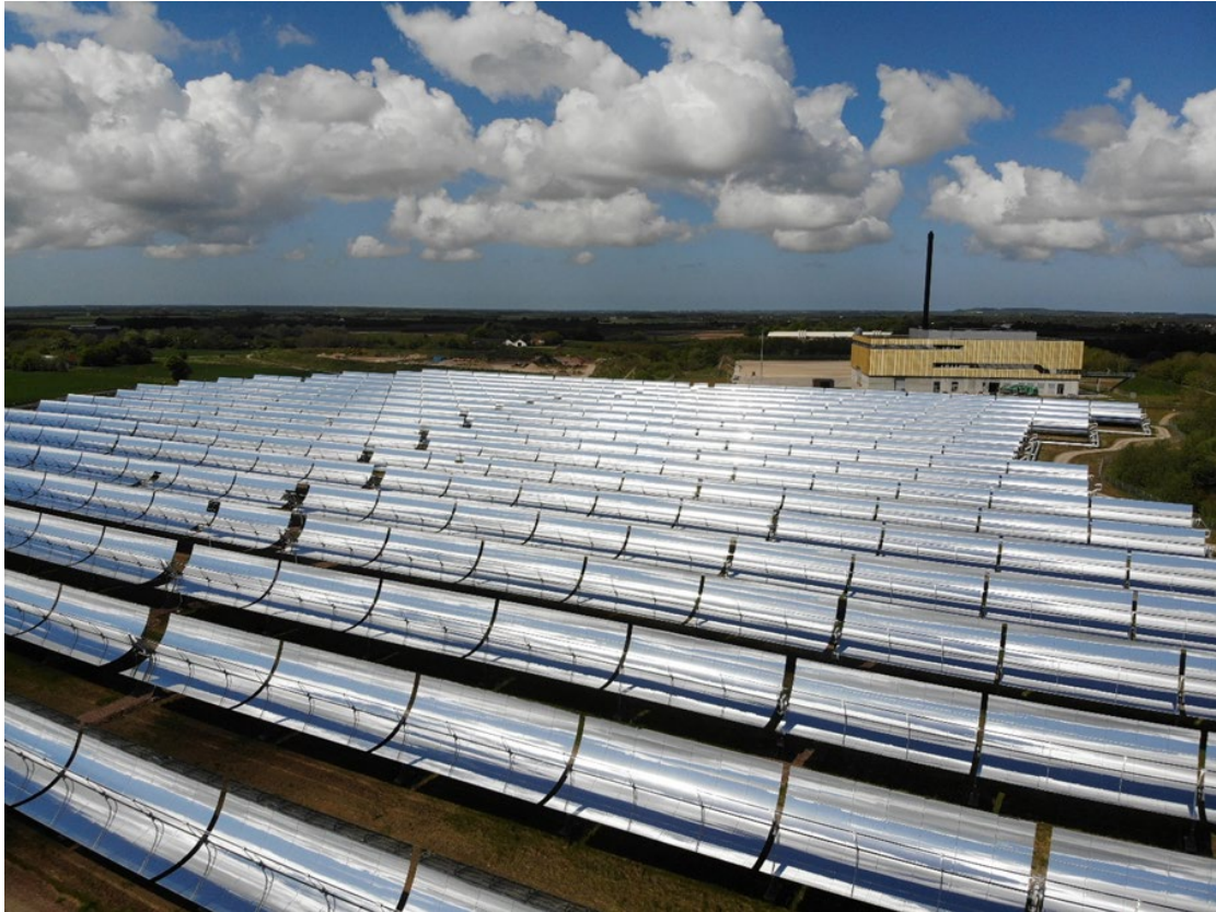
One axis tracking concentrating solar collectors at Brønderslev solar heating plant. The plant is used for both district heating and electricity production.(DTU)
