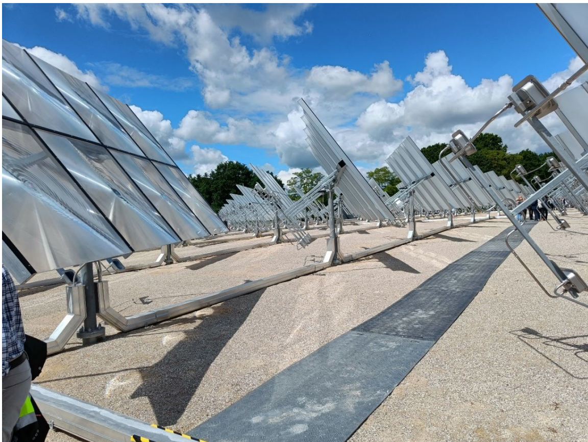
Two axis tracking concentrating solar collectors at Hørsholm solar heating plant. (DTU)
